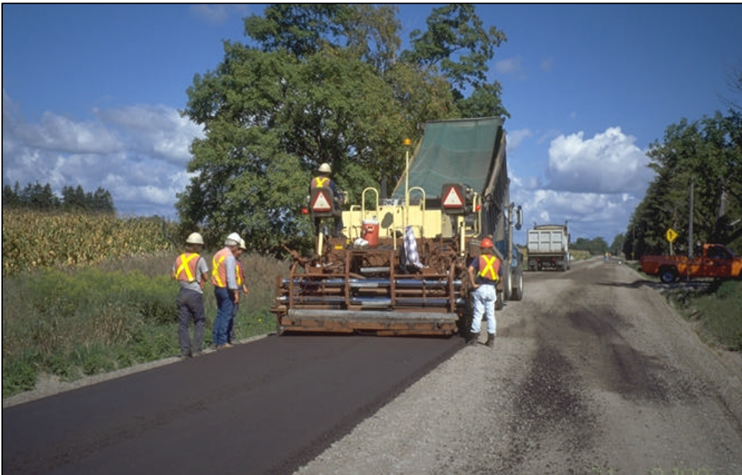
Figure 11 - Paving of Emulsion Stabilized Granular Material
