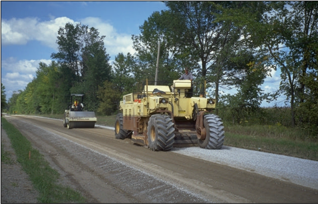
Figure 8 - Blending Operation of Corrective Aggregate with Existing Granular Material
