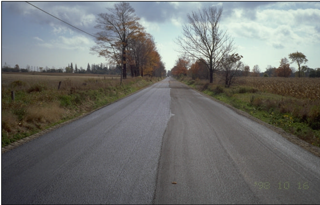
Figure 13 - Application of a Type II Slurry Seal Surfacing
