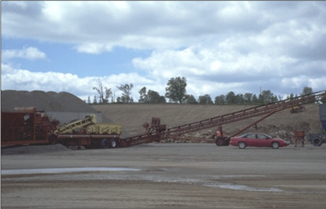
Figure 10 - Cold Mix Plant
