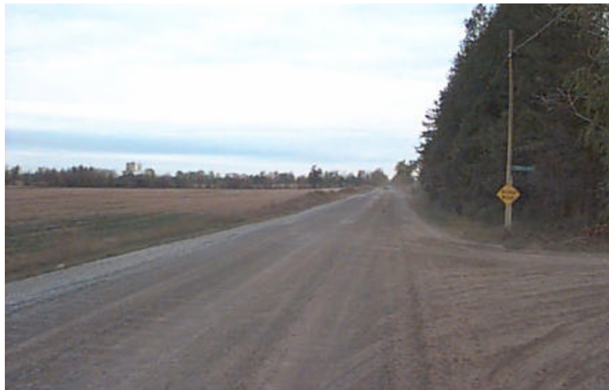
Figure 1 - Condition of York/Durham Line 30 before Pavement Rehabilitation
